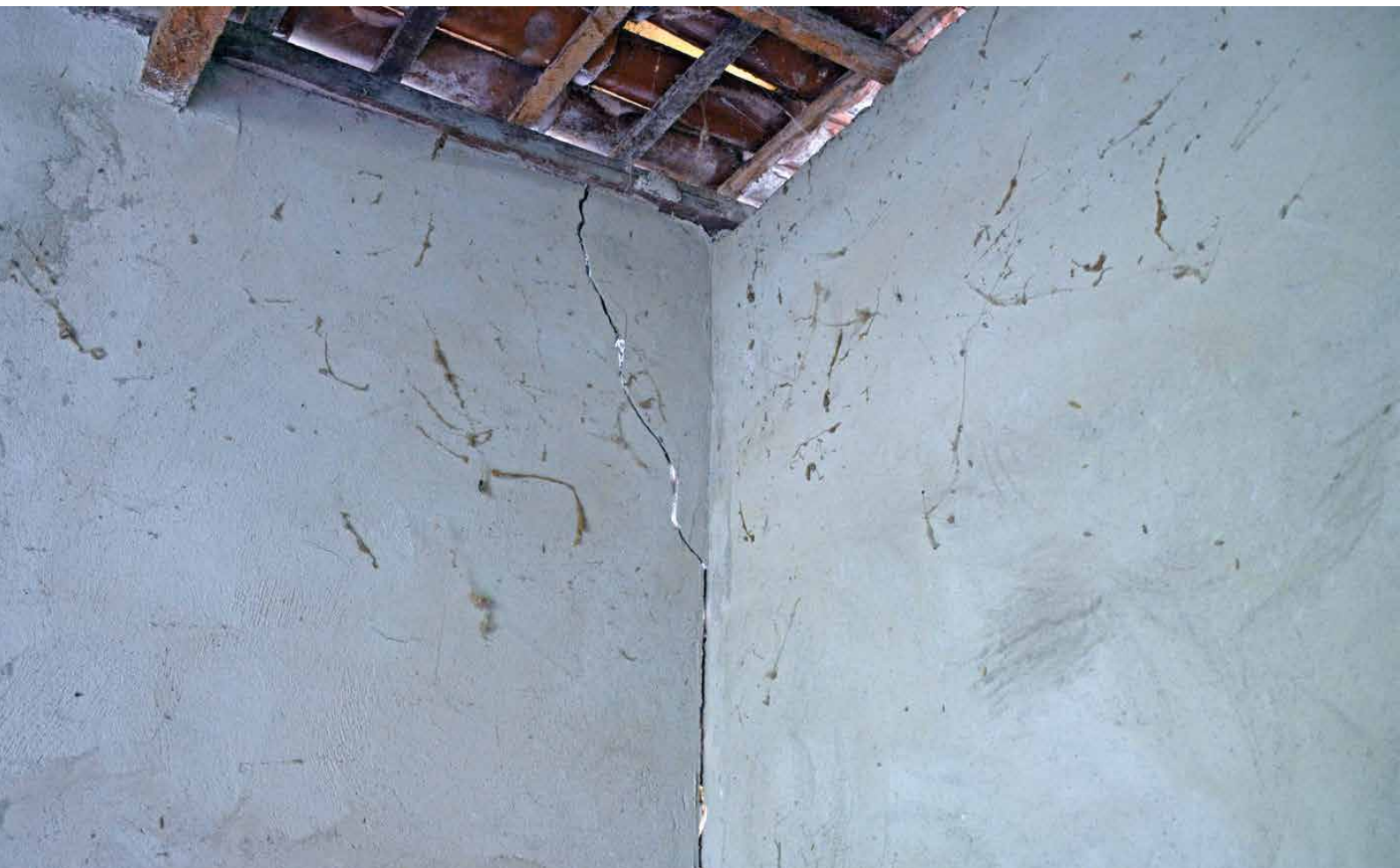
CRACKED WALL IN A HOUSE GIVEN BY TRAPICHE MILL TO A FORMER RESIDENT OF THE ISLANDS OF SIRINHAÉM. THE COMPANY PROMISED TO DELIVER ADEQUATE HOUSES BUT DWELLERS SUFFER FROM COLLAPSE RISK.
